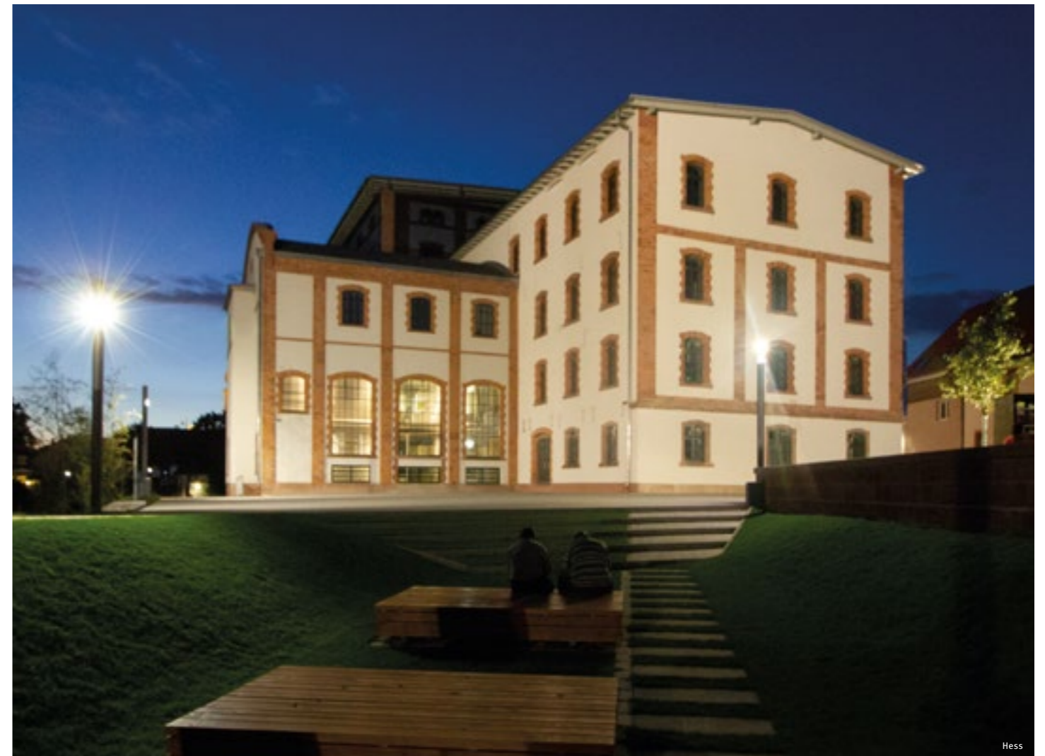
... and also at night. In the evening hours, the building which is elegantly staged, using projection technology, as well as the square as a whole convey a very comfortable atmosphere.
